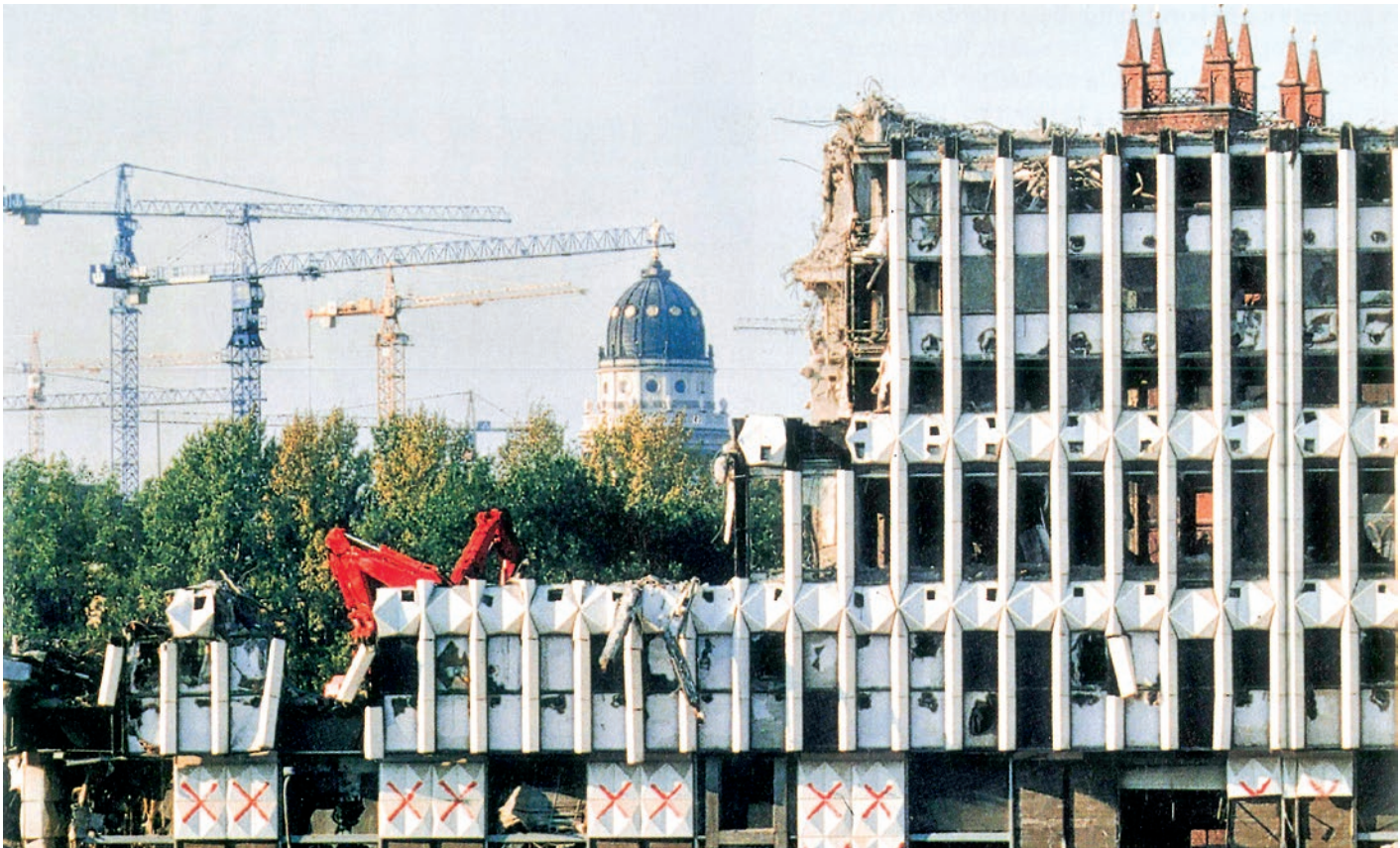
An example from history: When the former Foreign Ministry Building of the GDR was demolished, all the aluminium elements were recycled.
