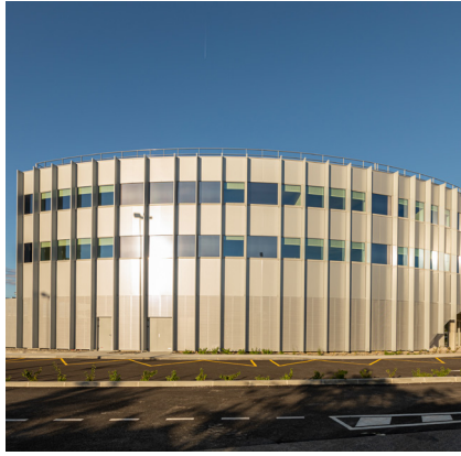
Terminal D Colomiers (31)
