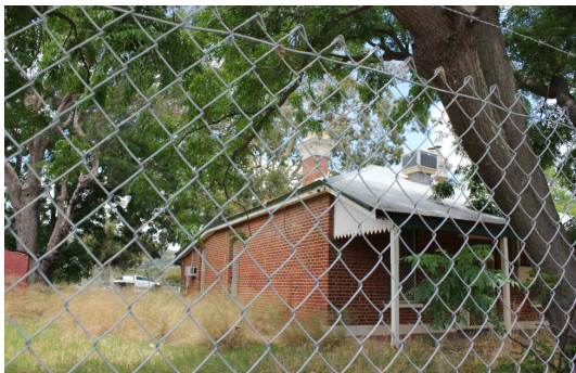
Face brick to the north elevation. Source: SCA 12/12/2018
