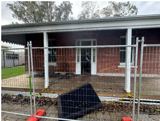
Figure 4 : Kelmscott Station Masters House west verandah.
