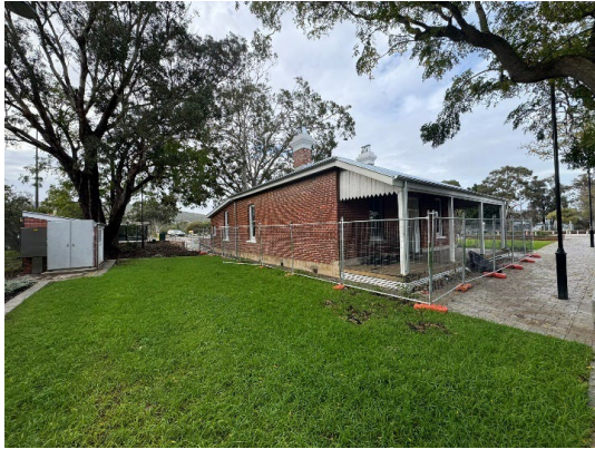
Figure 2 : Kelmscott Station Masters house north and west elevations looking south.
