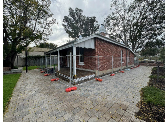
Figure 3 :Kelmscott Station Masters House west and south elevations looking north.
