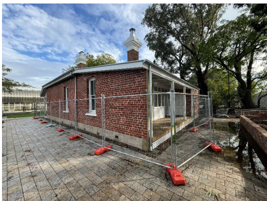
Figure 6 : Kelmscott Station Masters House east and south elevations looking north.
