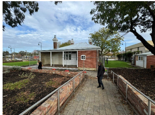
Figure 5 :Kelmscott Station Masters House east verandah.
