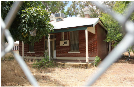
Symmetrical front verandah to the west elevation. Source: SCA 12/12/2018
