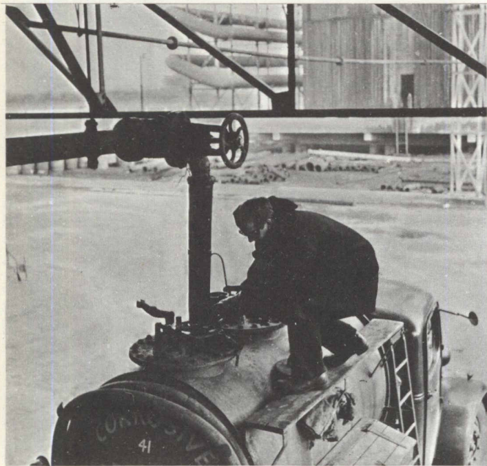
Sulphuric acid is generally transported in lead tanks. Laporte Industries Ltd.
