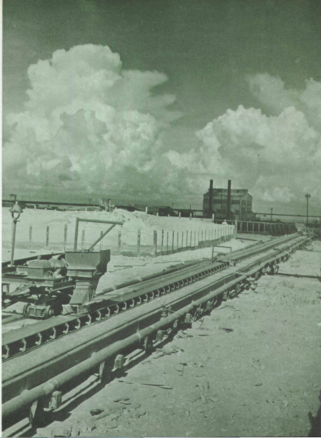
The sulphur mine at the Freeport Sulphur Company in Louisiana. The molten sulphur in the background is left to dry and solidify ; then it is cut into blocks for shipping. Radio Times Hulton Picture Library.
