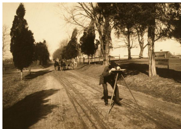
The tools of the trade have evolved, coming a long way since the days of the plane table soil survey pictured above.
