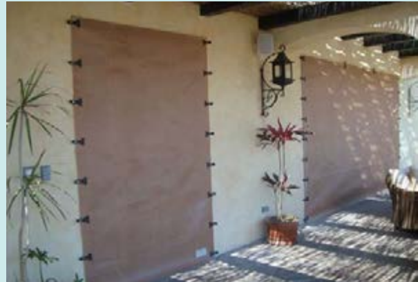
CH5-30: Homeowners fasten hurricane fabric that is fitted to window frames, a safety and time-saving measure that allows prompt evacuation.
