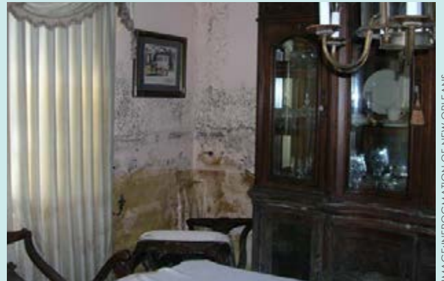
CH5-31: Lack of building ventilation can lead to mold problems in damp environments.
