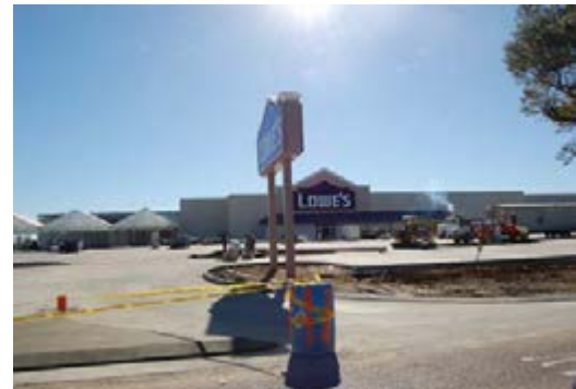
CH7-42: Stormwater facilities under construction.
