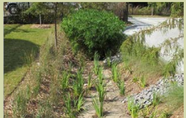
CH5-16: Bioswales provide pleasing landscape while capturing stormwater, helping it to absorb into the ground and clean the water.
