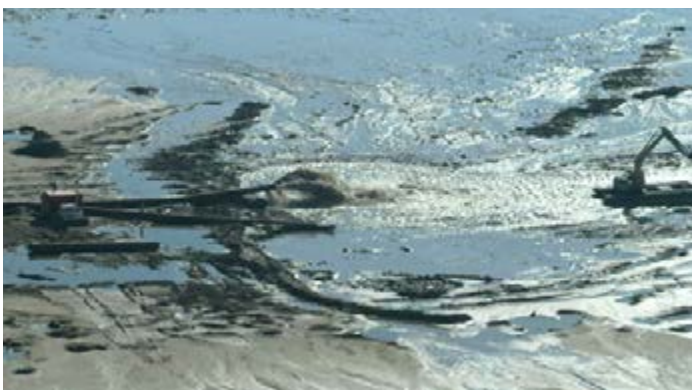
CH3-17: Dredged material from the construction of the West Bay Diversion channel is utilized to create new wetlands near the mouth of the Mississippi River.
