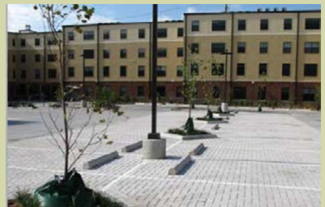
CH5-15: Pervious paving allows water to infiltrate on a site level. Because different areas have different soil composition, design needs to be site specific.
