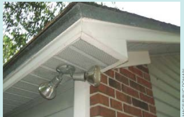
CH5-32: Soffits are some of the most vulnerable elements of a home and are susceptible to wind damage.
