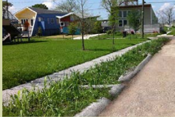
CH5-9: Residential roadway in Orleans Parish with stormwater curb extensions that absorb and treat runoff before it enters the drainage system.
