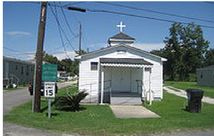
CH3-5: Phoenix, LA, a large African-American fishing community in Plaquemines Parish, was able to rebuild after Hurricane Katrina by leveraging limited resources and helping each other. The Zion Travelers Baptist Church and Community Center is a place for the community to gather and organize rebuilding efforts.
