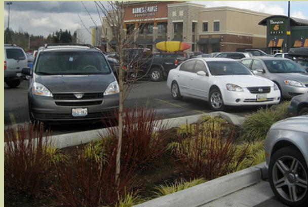
CH5-13: Bio-swales in parking lots can treat storm water on site through native vegetative plantings.
