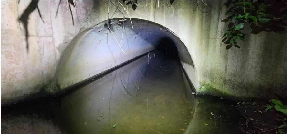
Figure 4. The larger culverts are more open but allow for fox and cat travel. This one had more water than the others but still showed no signs of Microbat presence during the visual inspections or Echo Meter Touch 2 monitoring.
