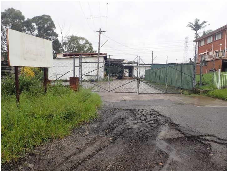
Figure 18. Survey Unit 1, view south showing previous commercial occupancy and concrete foundation
