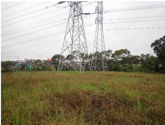
Figure 25. View south showing high voltage powerlines
