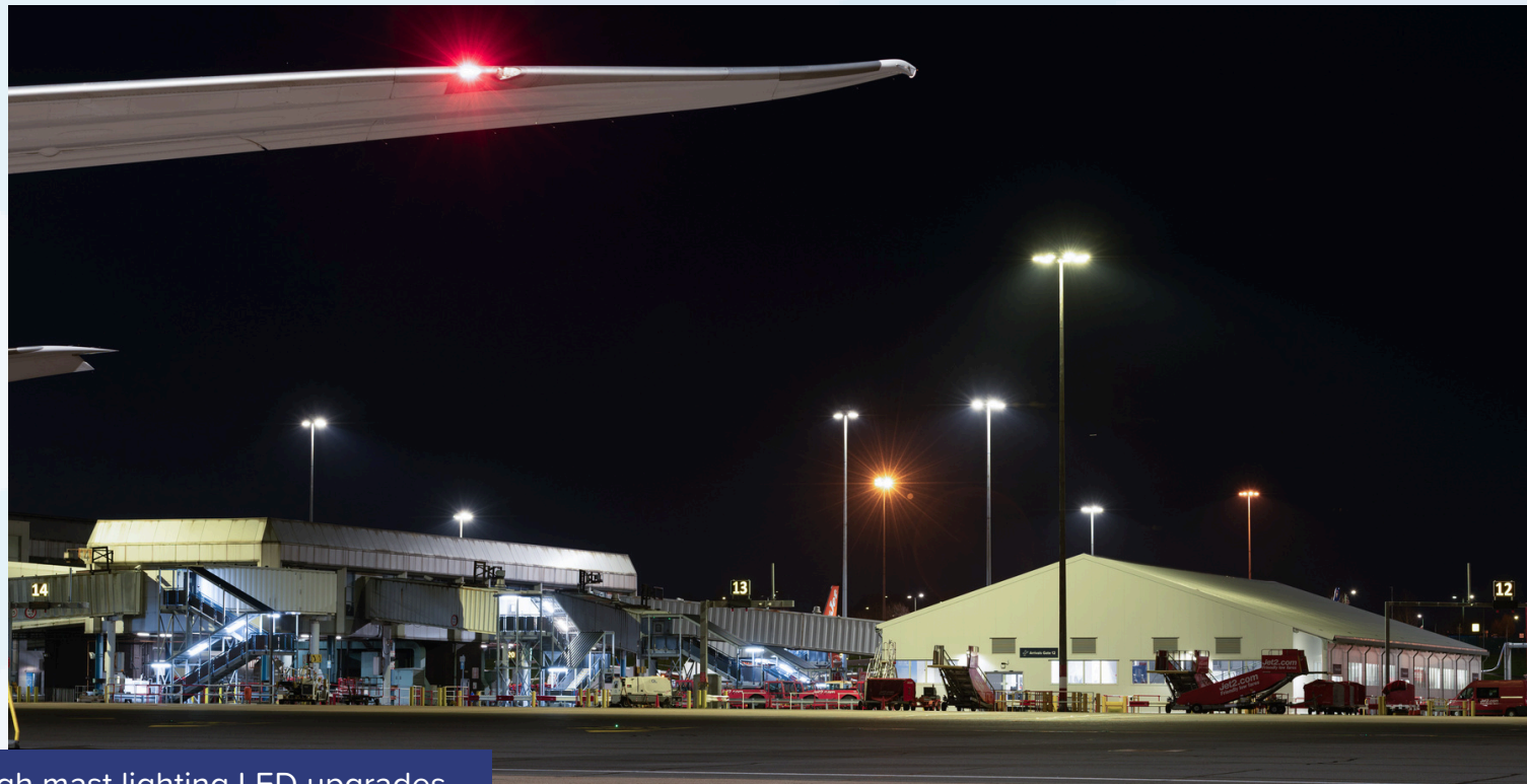
High mast lighting LED upgrades
