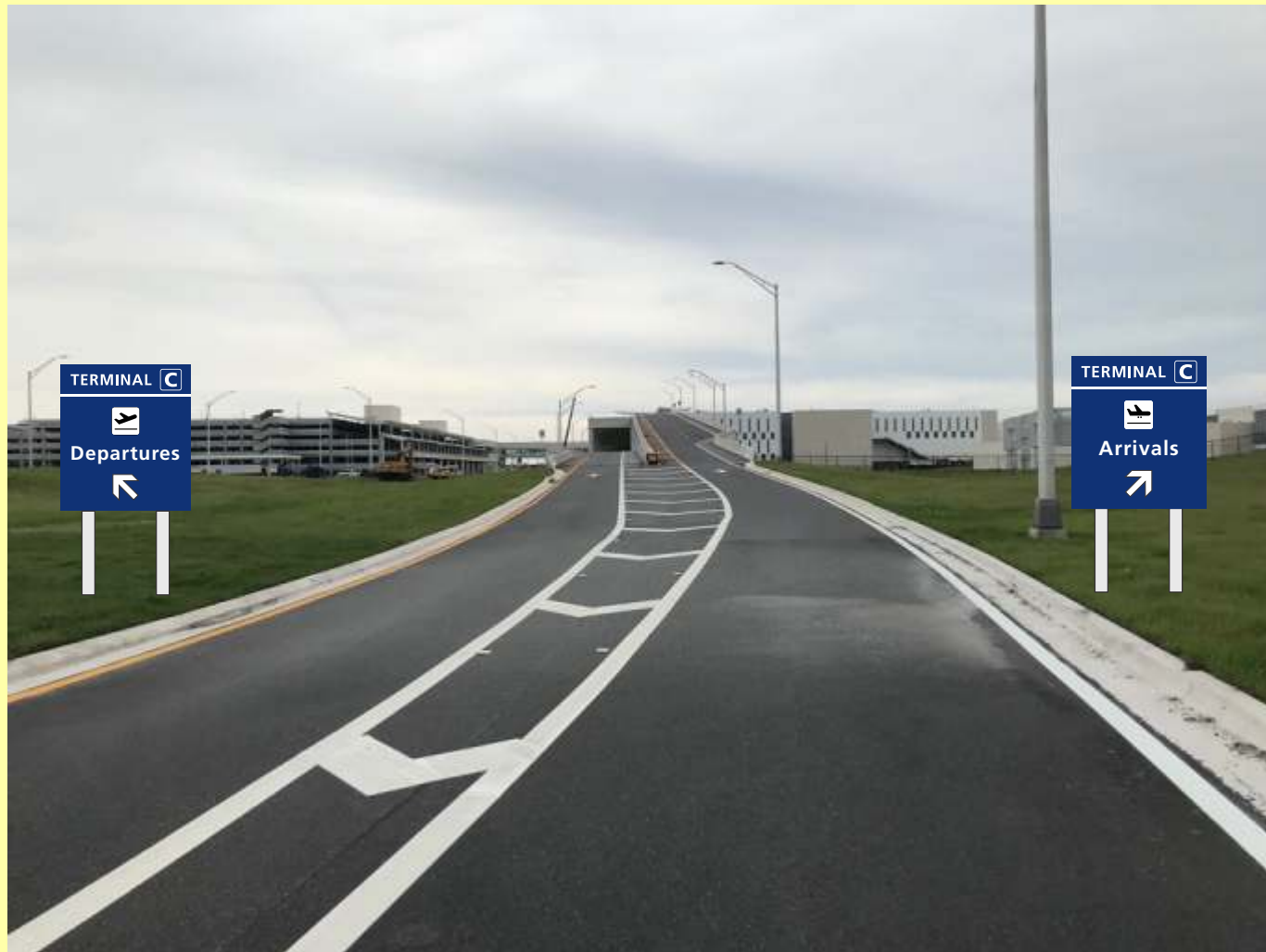
Roadway - Entry Area (looking South)
