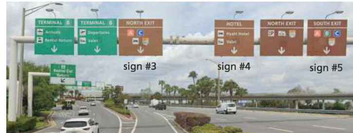
Existing Location View (structure #LB04)
