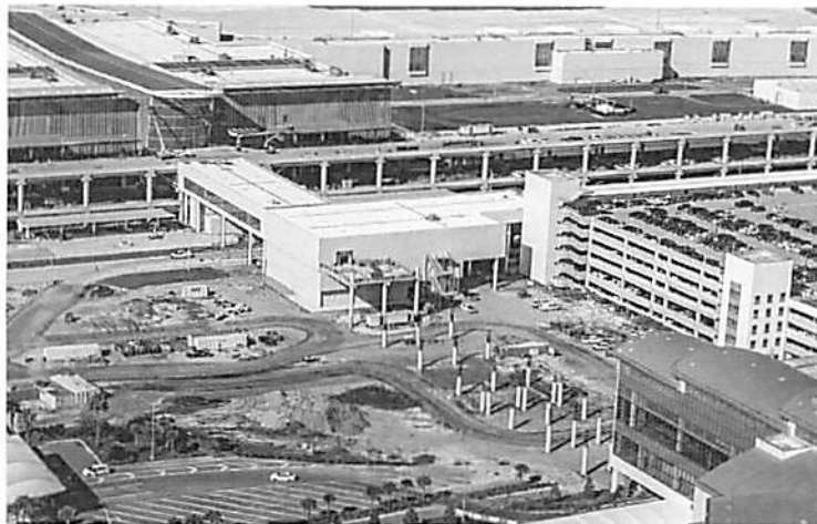
Existing STC GTF Pedestrian Bridge
