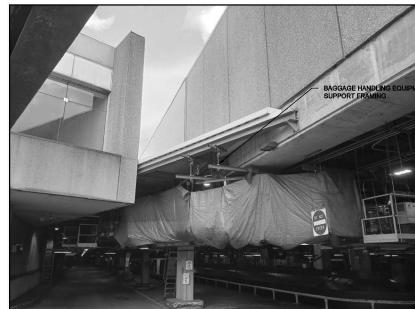
EXISTING METAL DECK ROOF EDGE TO BE ENCLOSED
