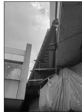
CONCRETE SOFFIT BEAM AT GRIDLINE '0.5'
