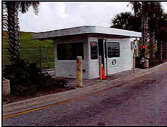
3) BLDG. #0856 GATE E-50 GUARD SHACK 116 S.F.
