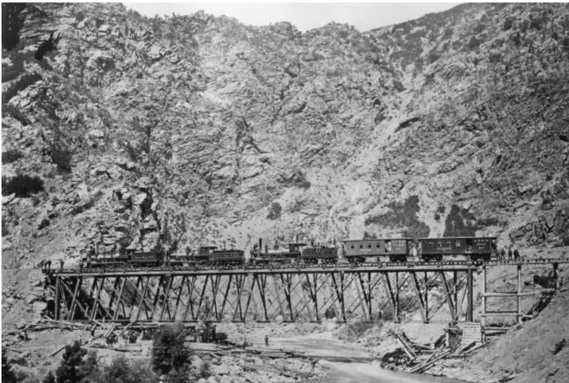
Construction of the Union Pacific section of the Transcontinental Railroad across Devil's Gate Bridge, Utah, circa 1869. PhotoQuest/Getty Images
