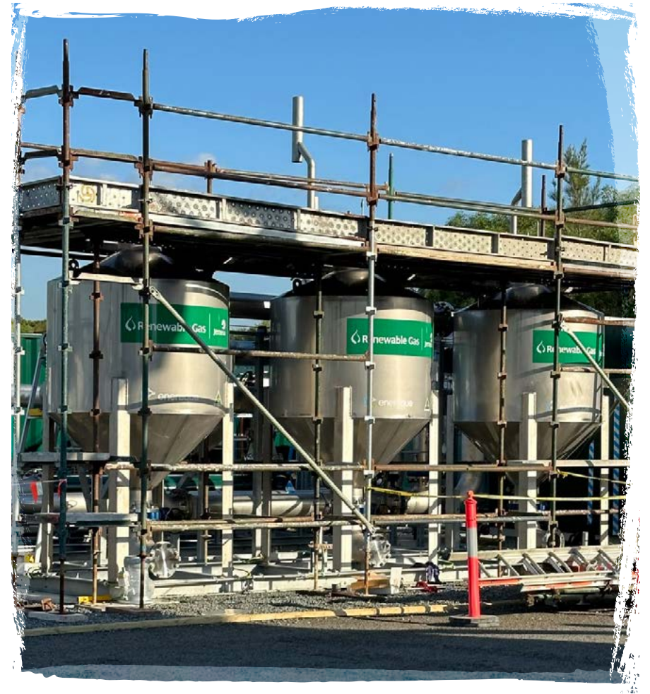
Construction of Australia's first biomethane-to-gas-injection project advanced in 2022
