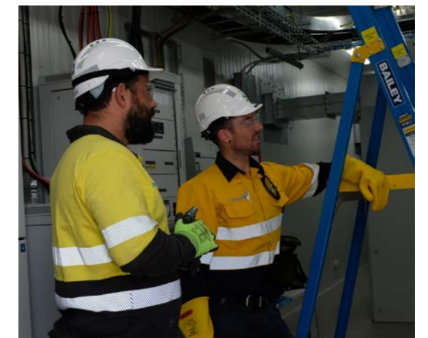
Our team members delivering data centre connections
