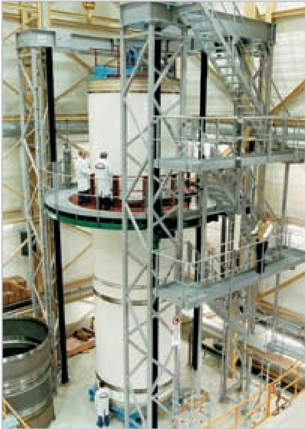
Installation of lifting system with flexible protection boots for approx. 9 m of lift.
