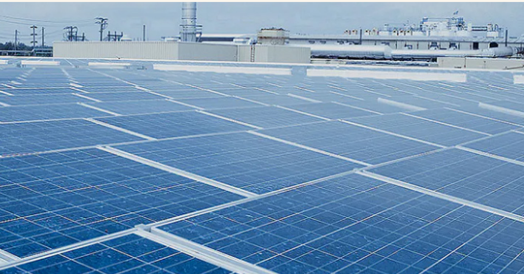
The 3.3 acres of 3,900 solar panels at our Salem, New Jersey facility generated 677,406 kilowatt hours to help power the site in 2023.
