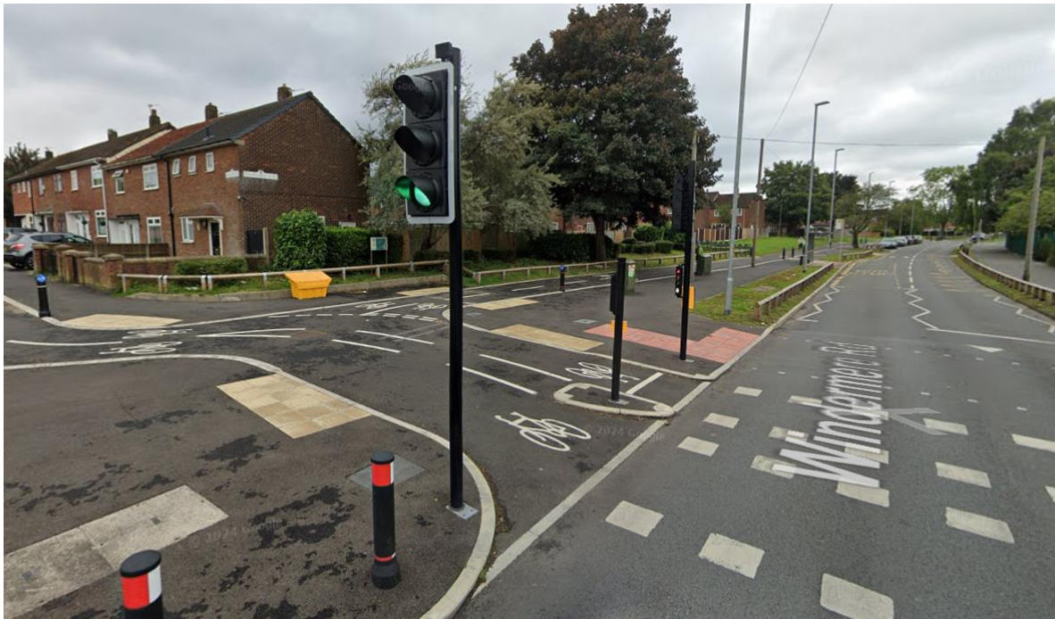
Figure 0-4 - Active Travel Infrastructure outside Bowlee Primary School on Windermere Road
