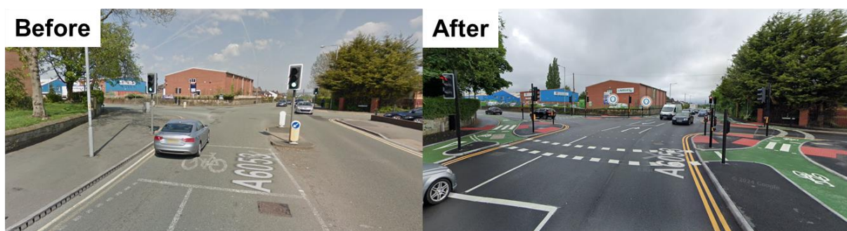
Figure 0-1 - Gladstone Road/Bolton Road Junction Redevelopment
