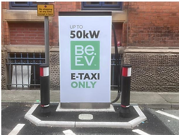
Figure 2-8 – Taxi Rapid Charging Point Installation
