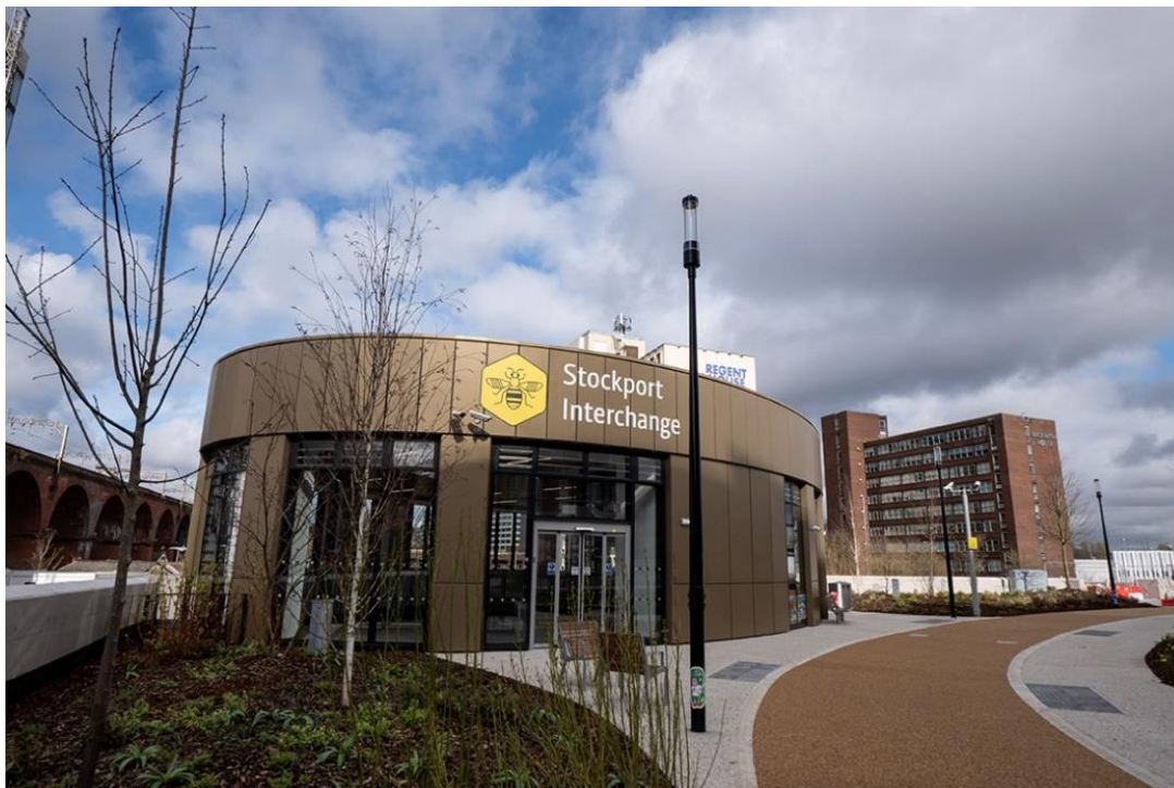
Figure 0-11 - Stockport Interchange viewed from Swaine Street
