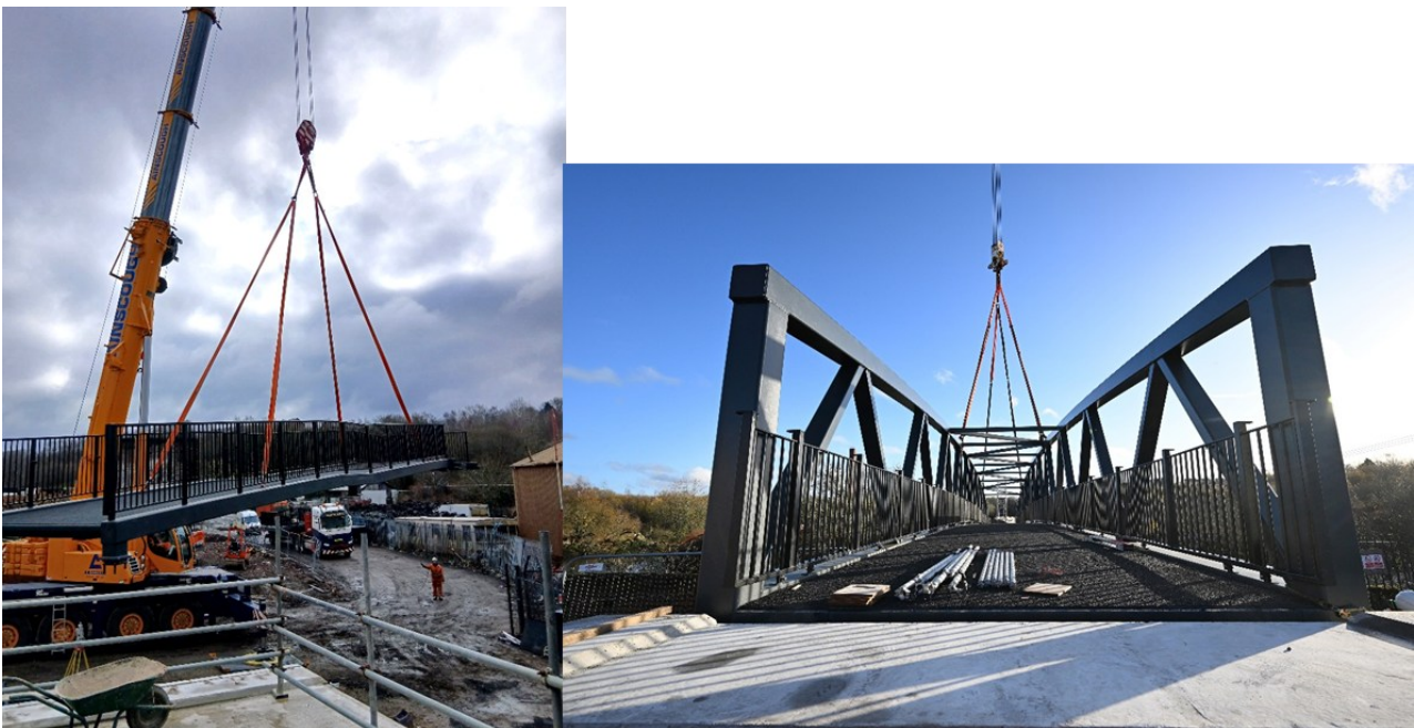
Figure 2-12 - Installation of the new Milltown Street Bridge
