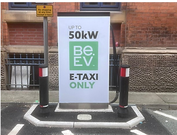
Figure 2-8 – Taxi Rapid Charging Point Installation
