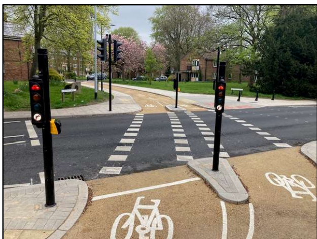
First completed Cyclops junction in Hulme, Manchester.
