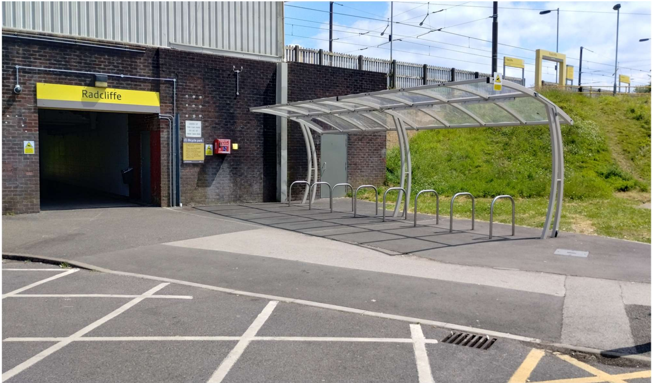
New cycle storage at the Radcliffe stop on Metrolink's Bury line.
