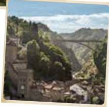
Galtertal bridge, Fribourg
