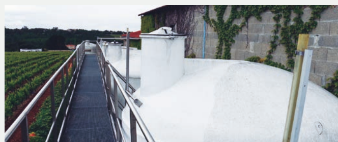
French winery Gennevilliers, France. ECO G 3-Pipe units. One of the best solution utilized our ECO G solution for wine production process.
