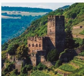
Gutenfels. Hotel. Kaub, Germany. Aquarea and Aquarea Smart Cloud.
