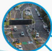
Ground access work
