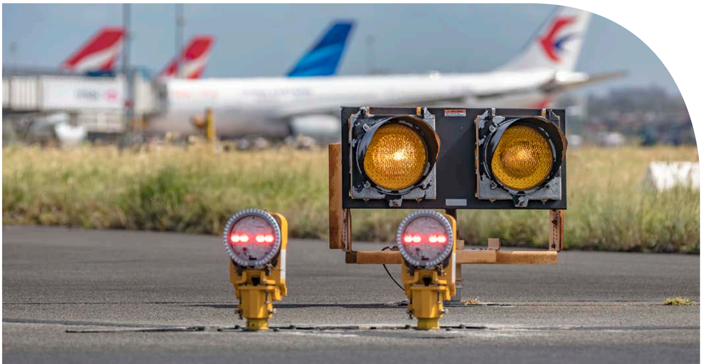
Image 9-8: Elevated stop bar lights and guard lights to help facilitate taxiing airfield
