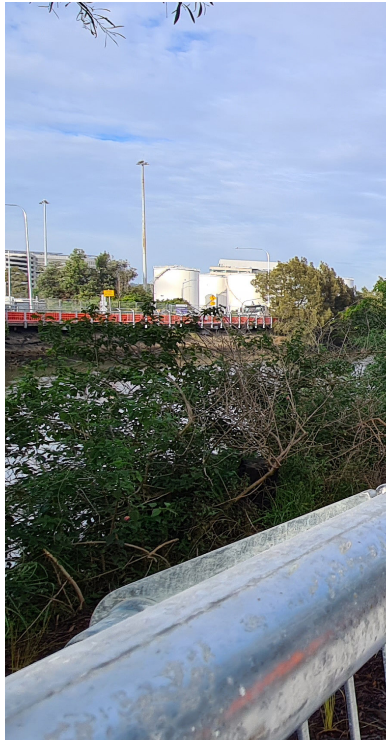
Figure 5: New shared path (north of Alexandra Canal)
