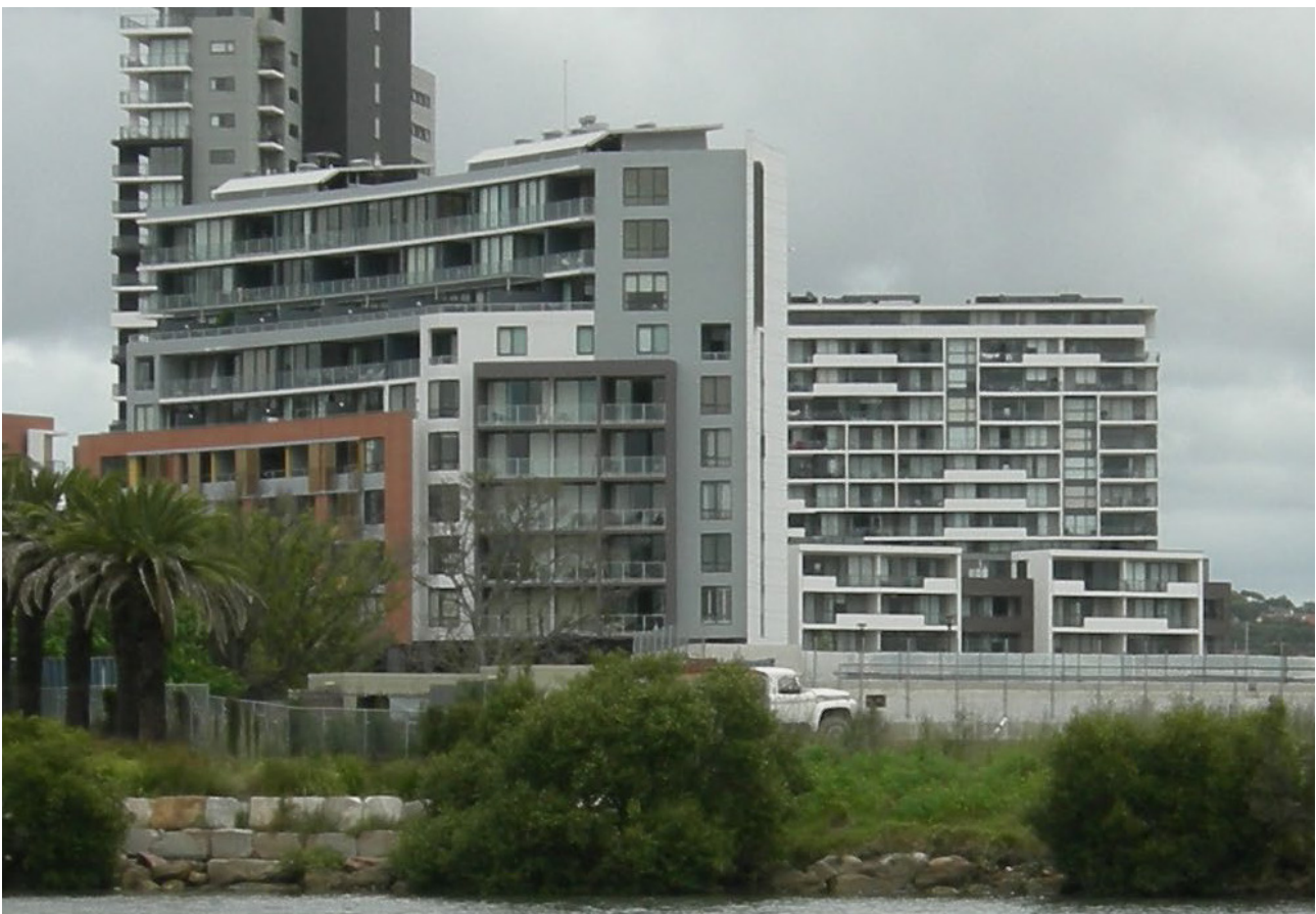
Figure 8: New development at Discovery Point, Wolli Creek
