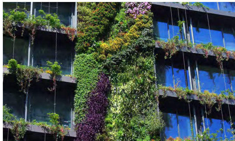
Figure 199. Vertical gardens and facade systems at One Central Park, Haymarket, attests to the potential for living walls to thrive in harsh conditions, and where maintenance access is restricted
