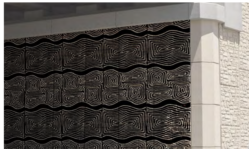
Figure 125. Examples of integrating Indigenous design into bridge abutment wall with colour and pattern
