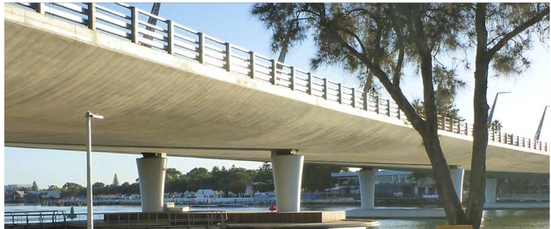
Figure 126. Refined superstructure with integrated parapet, Mandurah Bridge, Western Australia
