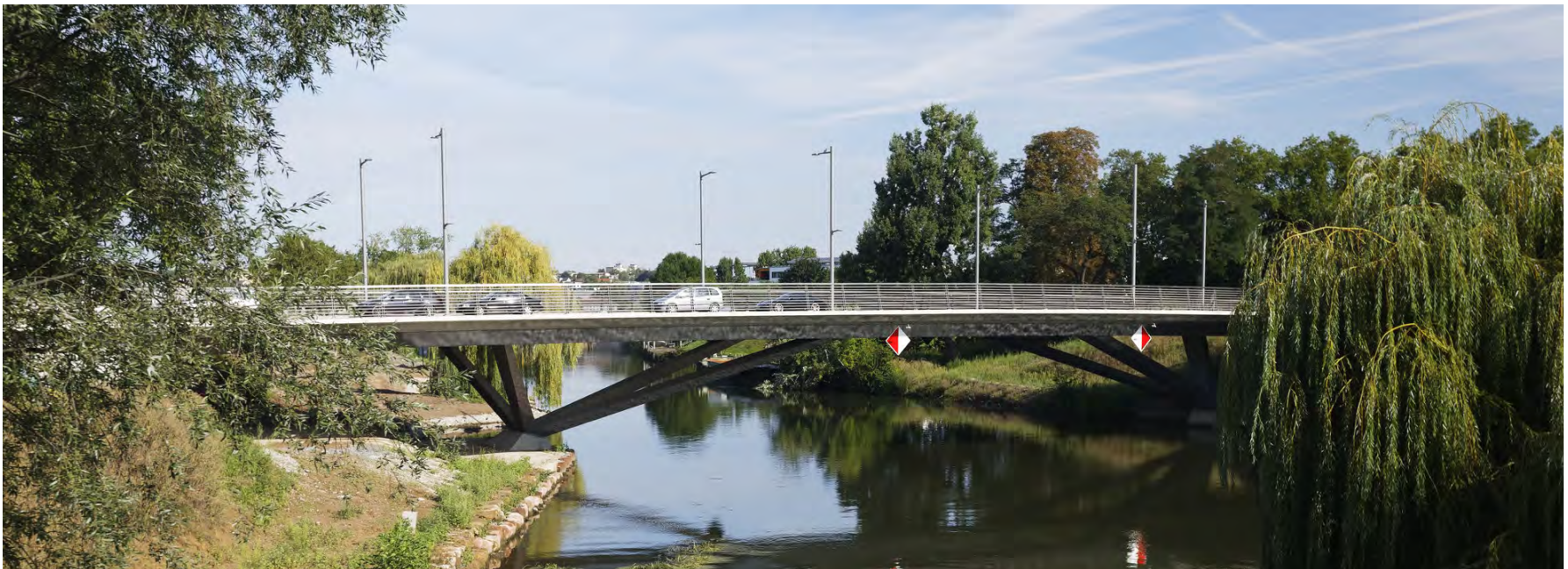
Figure 132. Bleichinselbrücke, Heilbronn, Germany has a minimal superstructure and visually light fencing
