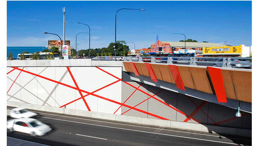
Figure 135. The Gallipoli Underpass in Adelaide is a good example of the use of striking colour and of integration between the parapet and wall design
