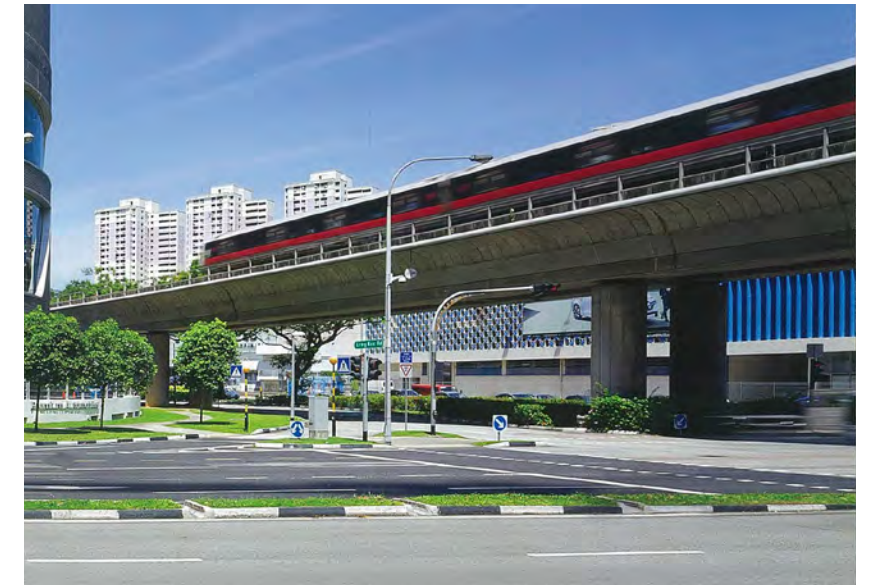
Figure 139. The viaduct at Singapore airport provides a good example of a refined and elegant soffit
