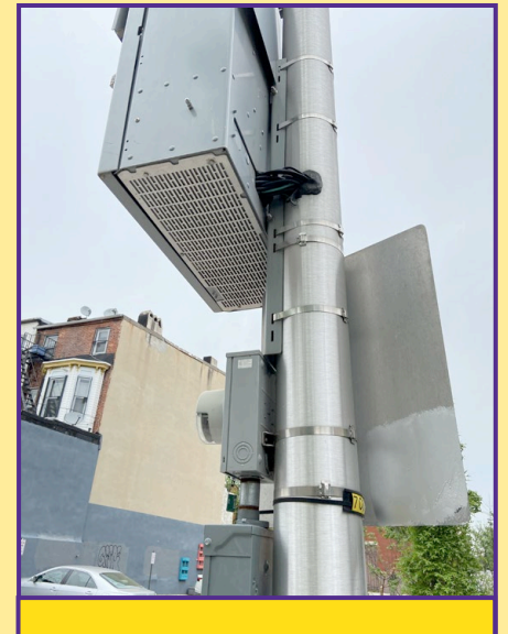
Wireless infrastructure attached to DOT pole with below-ground conduit
