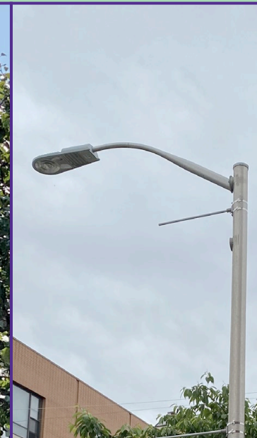
Aluminum roadway pole with LED fixture (new)
