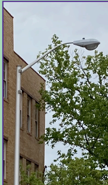
Aluminum roadway pole with HPS fixture (old)
