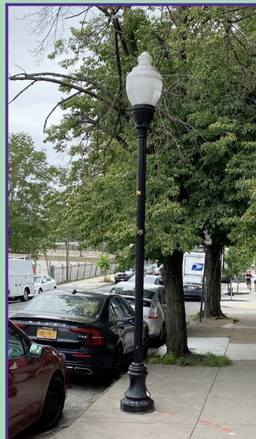
Pedestrian post with acorn top (LED or HPS)
