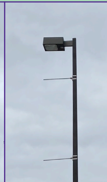
Steel roadway pole with HPS fixture (old)
