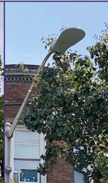
Aluminum roadway pole with Bmore Bright LED fixture (new)
