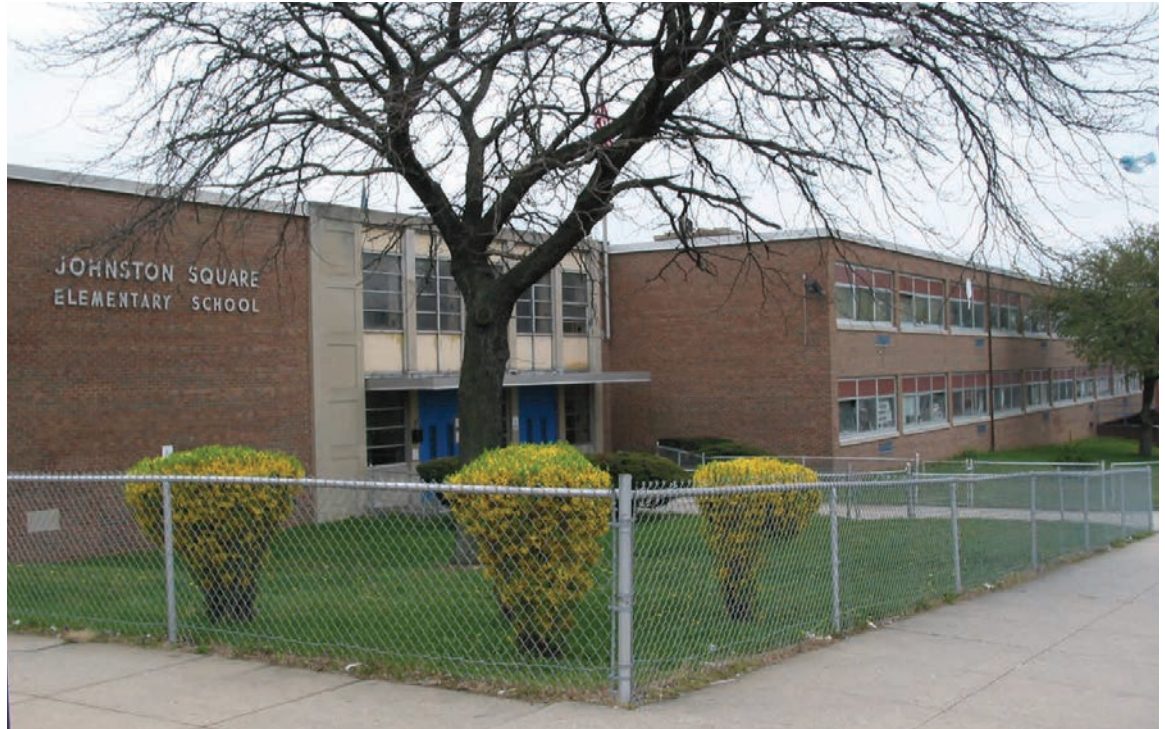
Johnston Square Elementary School, Valley Street
