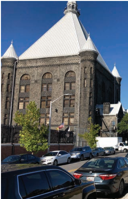
City Jail Roof Line
