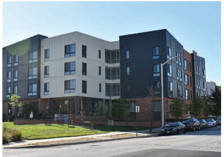
Lillian Jones Apartments- New Multifamily Housing
