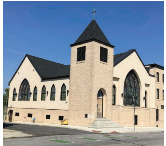
Mt. Sinai Church Refurbished Facade (photo by Lil Trottman)
