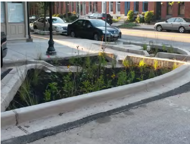
Curb extension planted for stormwater, Butcher's Hill, photo by Jared Barnhart
