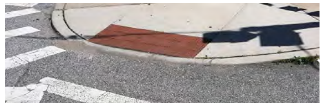
ADA compliant ramp, Baltimore, photo by Ross Hackett
