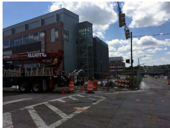
Construction at Coppin State Campus, photo by Ross Hackett
