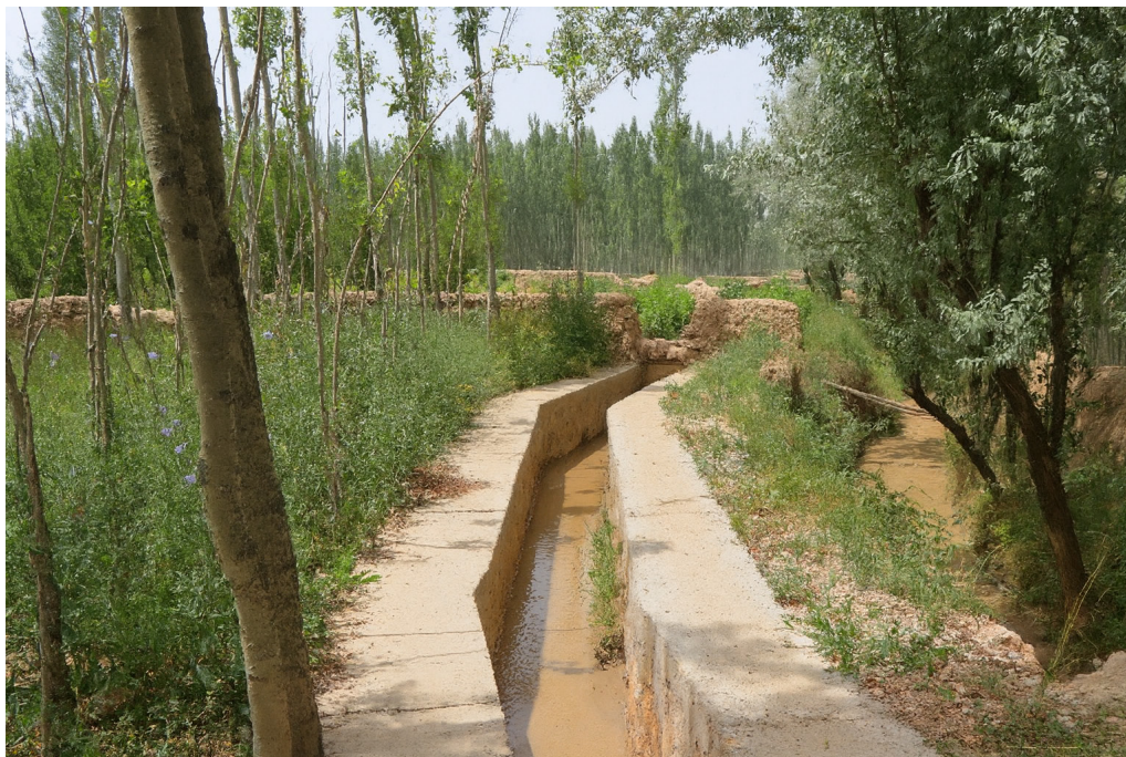
Irrigation canal in Samangan Province, Afghanistan.
