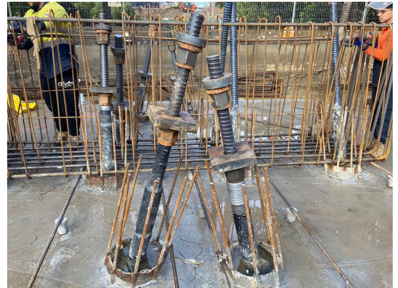
ALFRED STREET PEDESTRIAN BRIDGE, SYDNEY DCP MICROPILES
