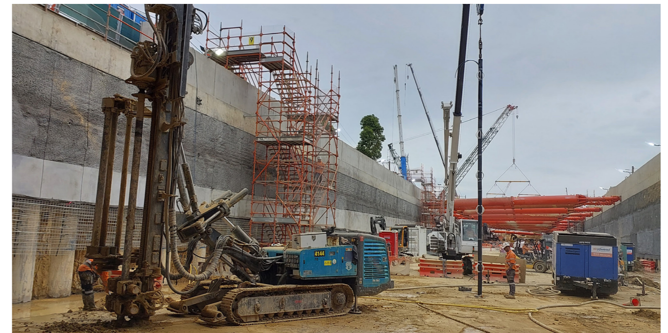
UNION ROAD, AUSTRALIA INSTALLATION OF MICROPILES
