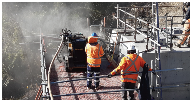
SMART ANCHOR DRILLING
