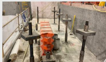
The Melbourne Metro Project is a 9 km twin TBM tunnel with five new stations across the central business district. DYWIDAG worked on the project from design to installation, providing technical advice, manufacturing, and supplying more than 1,000 strand anchors and 1,000 permanent pre-grouted DCP micro piles against hydrostatic uplift of the station boxes, and GFRP and High-strength Threadbar® Systems. DYWIDAG was recognized as a quality manufacturer and supplier.
