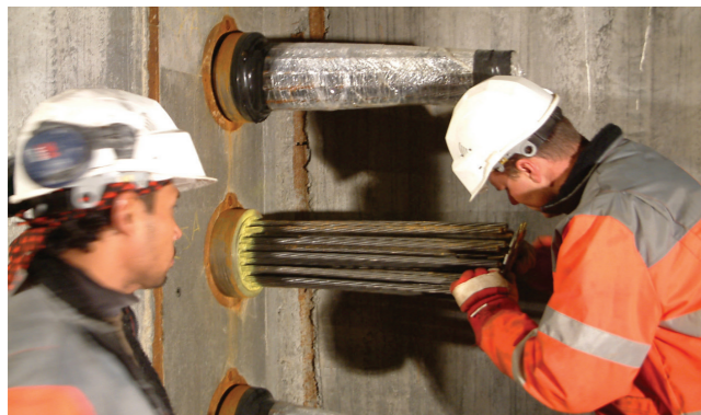
PT TENDON INSTALLATION
