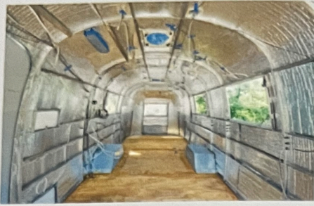
Removing the interior aluminum skin allows new wiring and insulation.
