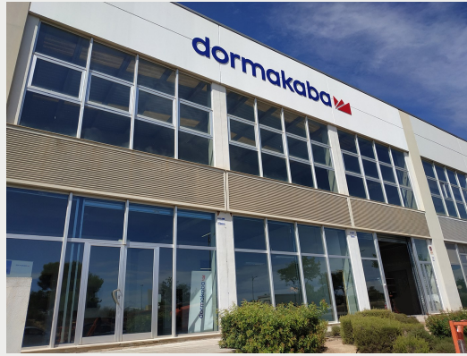
A dormakaba facility in Spain
