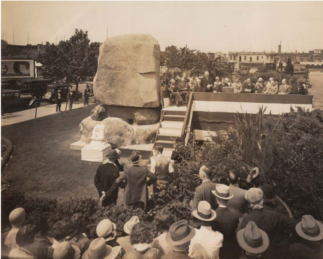
On April 26, 1930 a memorial honoring the professional contributions of Theodore Judah was commemorated in front of the Southern Pacific passenger station in Sacramento, championed by W.H. Kirkbride, M. ASCE, Chief Engineer of the Southern Pacific Company, seen above standing on the dais constructed for the event (Galloway Collection Colorado Railroad Museum).
