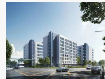
Production Center II 45000 m 2
