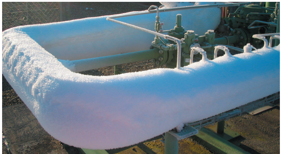
Icing of a gas pipeline.
