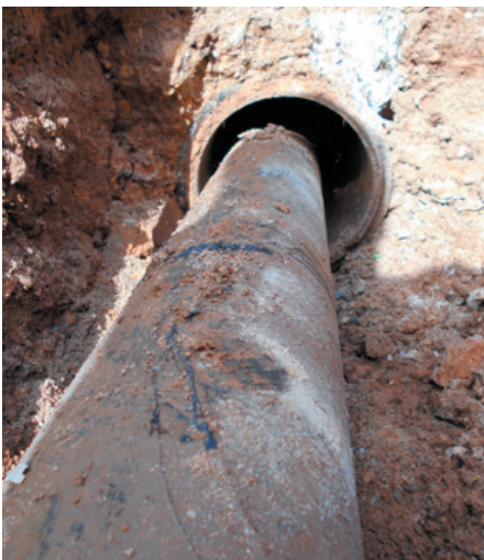
Pipeline running into a duct.
