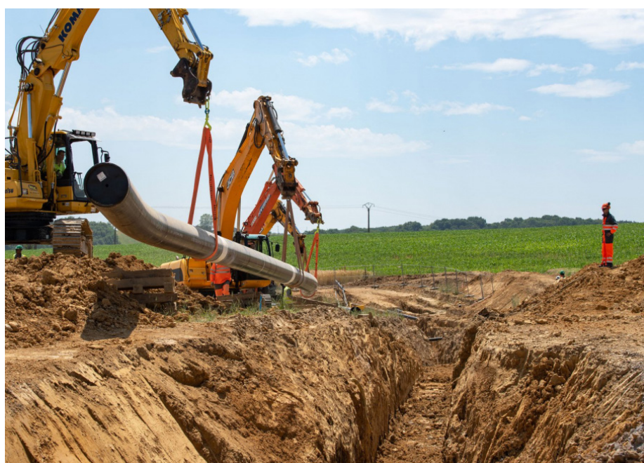
Laying a pipeline on a worksite.
